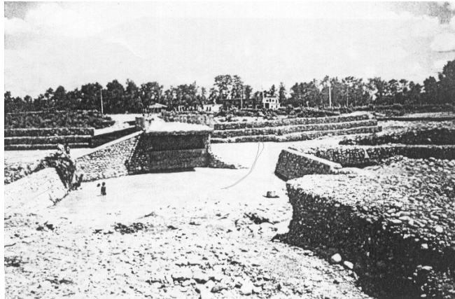
Fig. 7 Outflanking of a vented causeways on the stream 'Danab Khola' in Nepal
