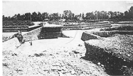
Photograph-1: Outflanking of a vented causeway due to restriction of waterway on the stream 'Danab Khola' in Nepal
