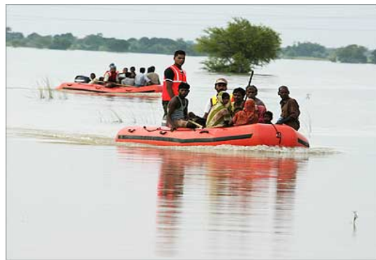
Photograph-3: Devastation brought about by river Kosi due to change of its course on August 18 th, 2008 due to Breach in left Embankment about 12 km upstream of Kosi Barrage
